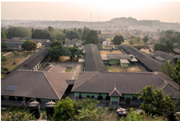
Das Sacred Heart Hospital in Abeokuta, Nigeria
